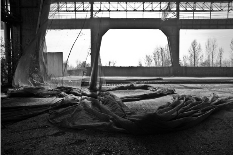
Figure 5: Falck Concordia inside view (Photo: U. Gillio 2015)
